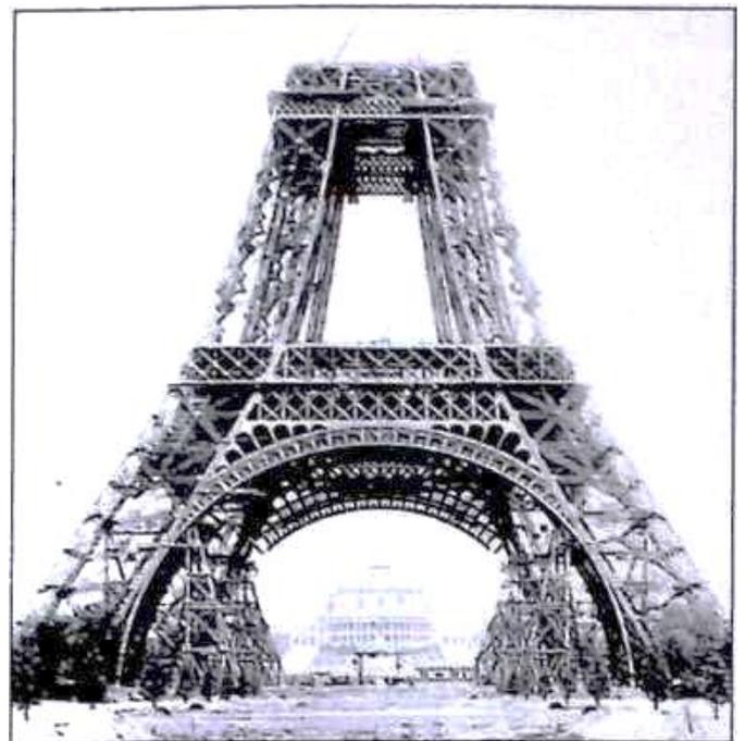
Figure 2.3.2: The Eiffel Tower under construction, 1888
